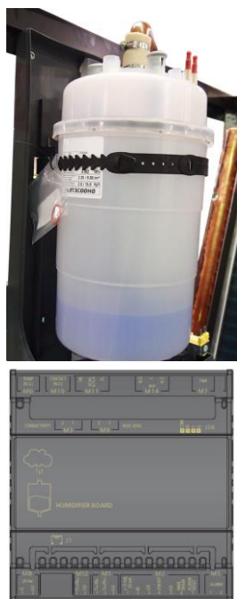
Humidifier control board
